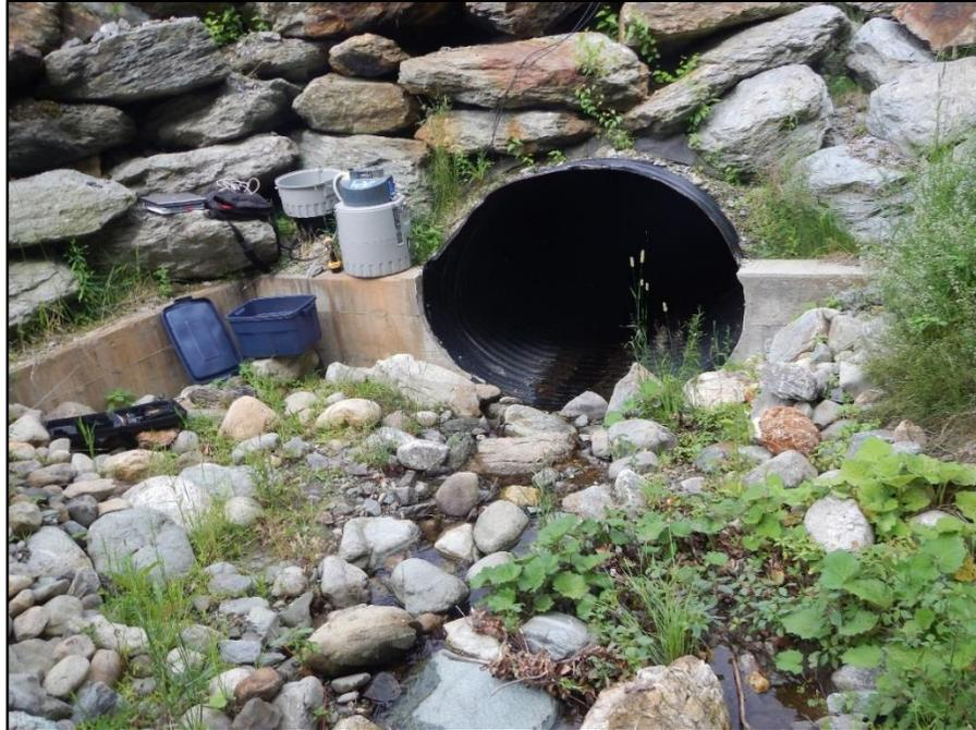
**Photograph 2. Automated sampler at Access Road culvert inlet, upstream from LS-A9 vegetated buffer area (VHB, 07/08/16)**
